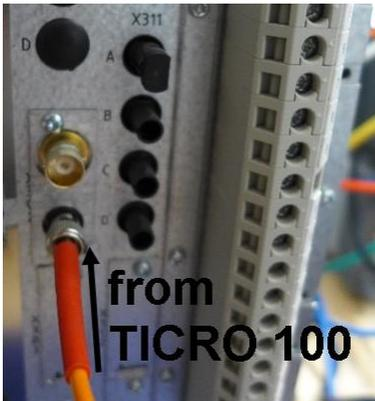
Figure 3: Time Synchronization Input of RET670
